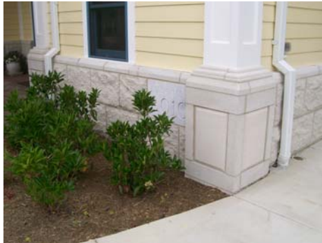
Masonry base & cement board siding
